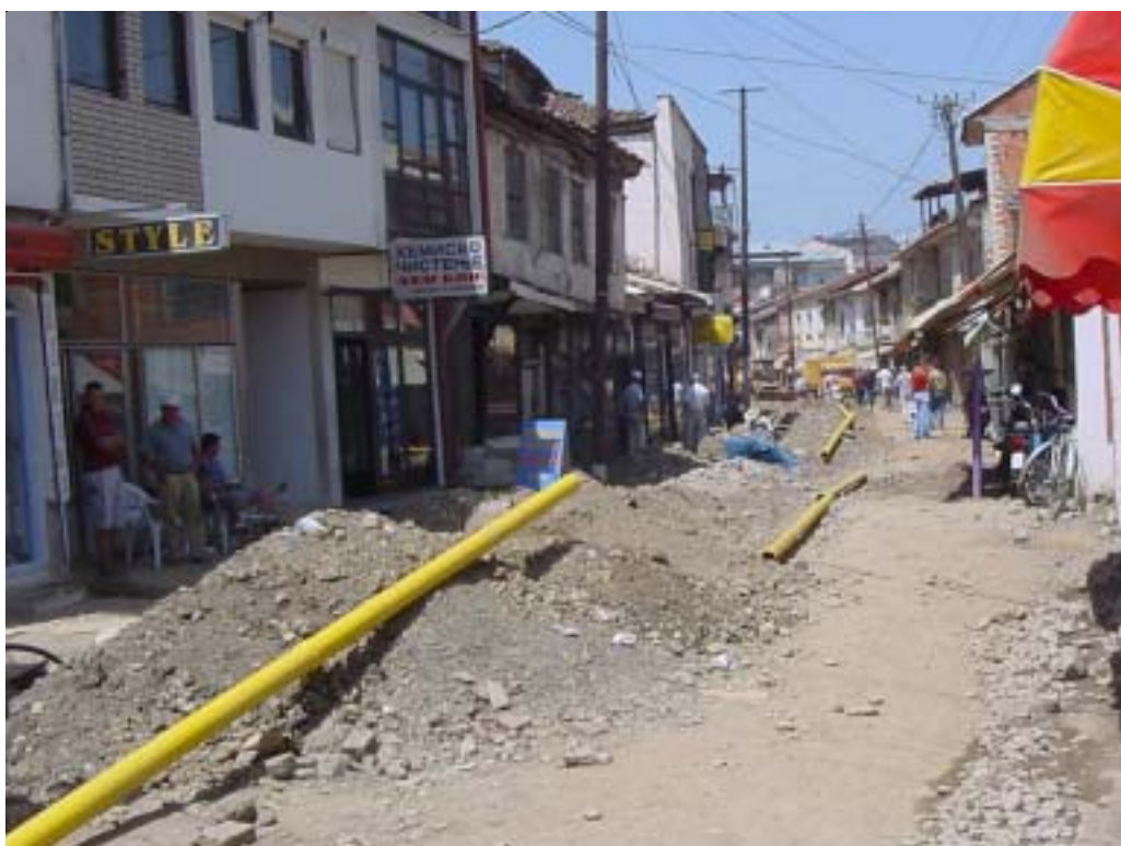
The sewer line is extended in the town of Ohrid.
