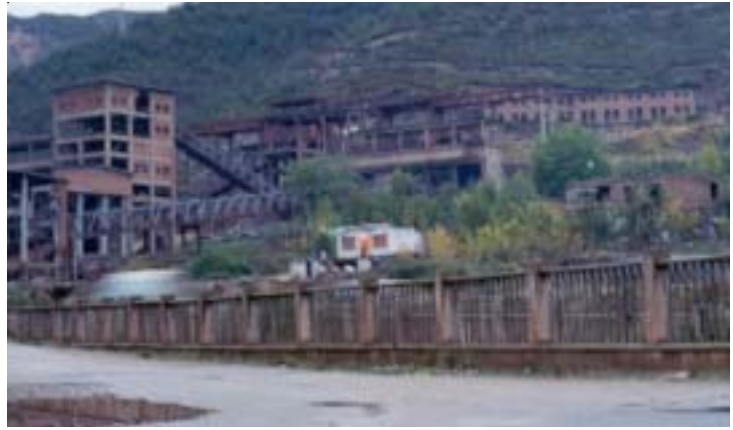
An abandoned mine along the south shore of Lake Ohrid in Albania may still be polluting lake waters.
